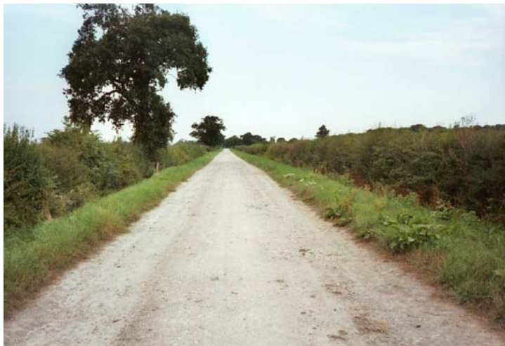
Fig. 5.4 Ardington Lane, Ardington is a typical enclosure road, looking more as it would have in the nineteenth century because today it is a bridleway and chalked. The road is 40 feet wide, ditched and hedged on both side and almost completely straight. The road with its verges was wide enough to allow various paths through when the road was wet and muddy.
